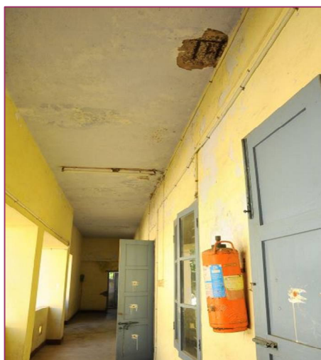
Exhibit 2.23: Damaged roof and time expired fire extinguisher
