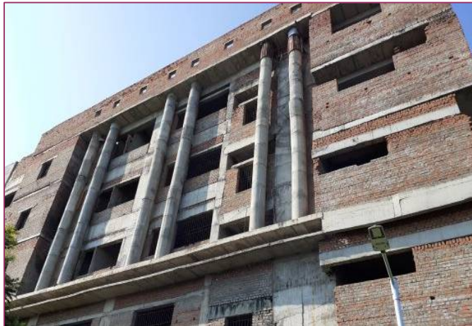
Exhibit 2.20: Facade of the incomplete building
